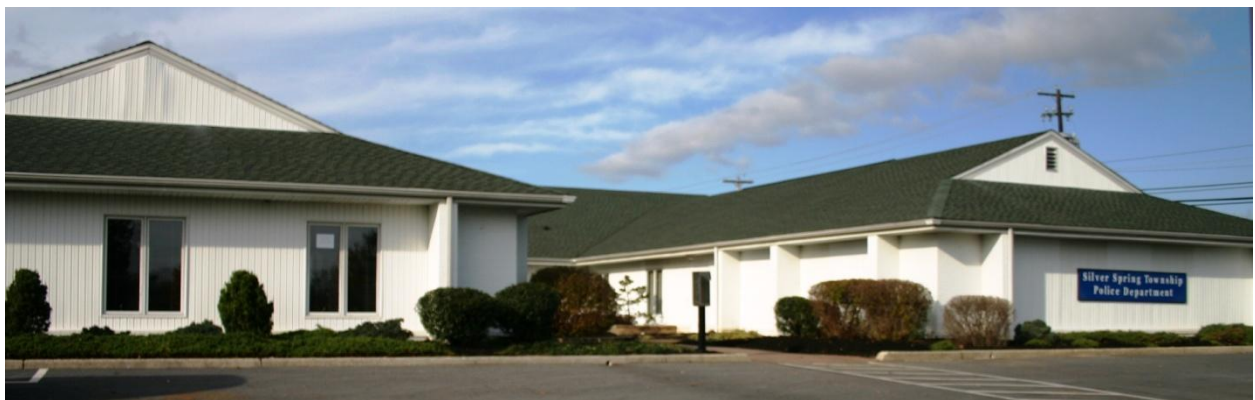
NEW POLICE / PARKS & RECREATION /SILVER SPRING TOWNSHIP SEWER AUTHORITY BUILDING
